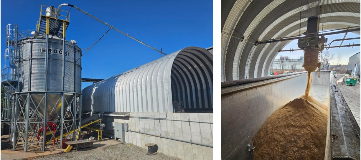
Figure 6: silo and truck-loading station
